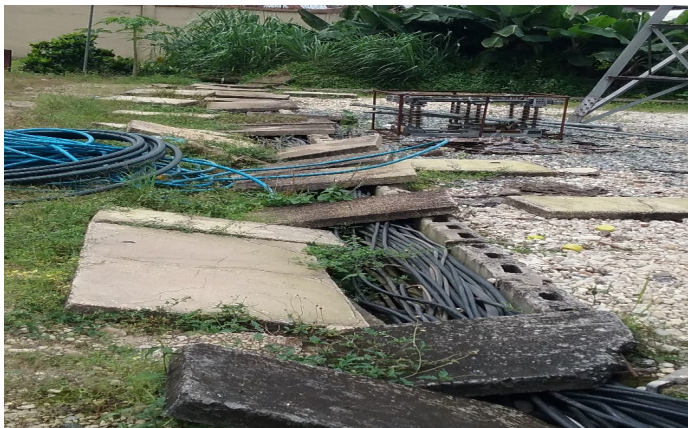
Figure 34: Broken/Collapsed trench cover slabs within the switchyard (posing potential injury risks Transformer Oil drums lying on the switchyard floor)
