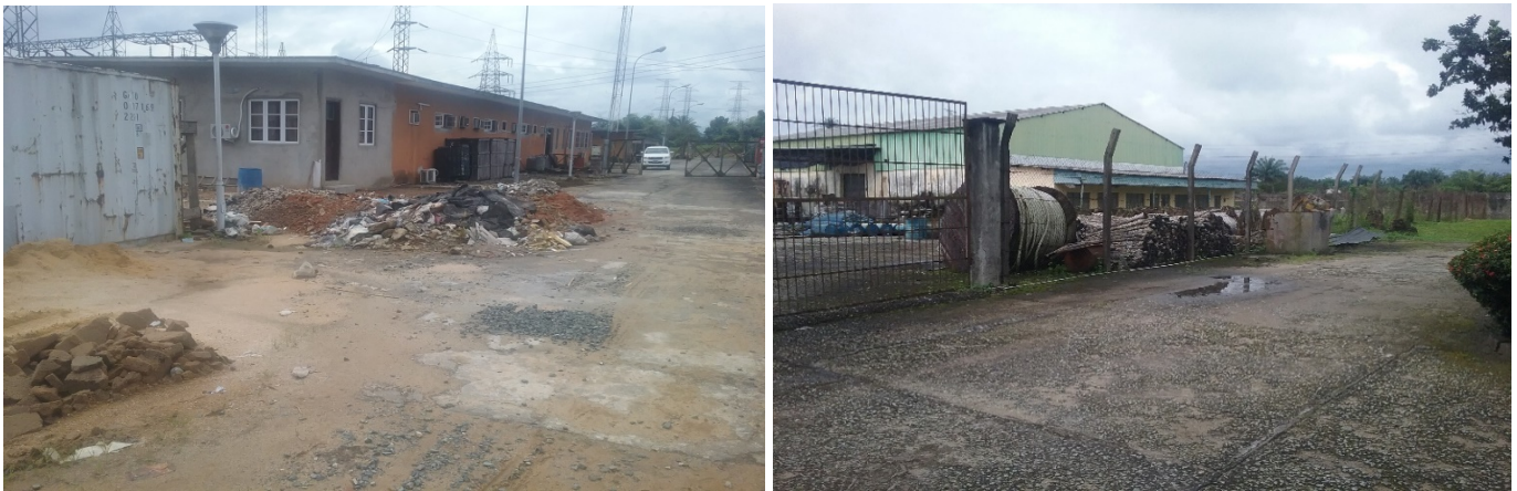
Figure 15: Extension works on-going on existing Control Room building /Well defined and fenced storage area the substation premise.
