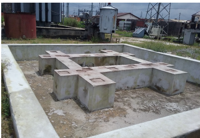
Figure 35: Transformer Plinth/Spilled oil from very old transformer(posing risks of ground-water pollution through seepage).
