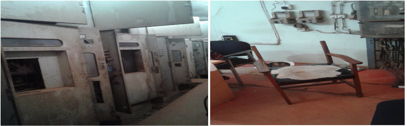
Figure 18: Old control Panels in Control room (ready for decommissioning)/Decrepit furniture being use by operators.
