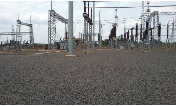
Figure 51: Properly maintained Switchyard floor/(well- gravelled and free of grasses or shrubs)/ Trench cover slabs intact, protecting power cables (eliminating the risks of accidental shock/electrocution).
