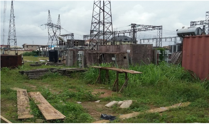
Figure 32: Overgrowths within the Substation premise/Improperly stored transformer oil drums.
