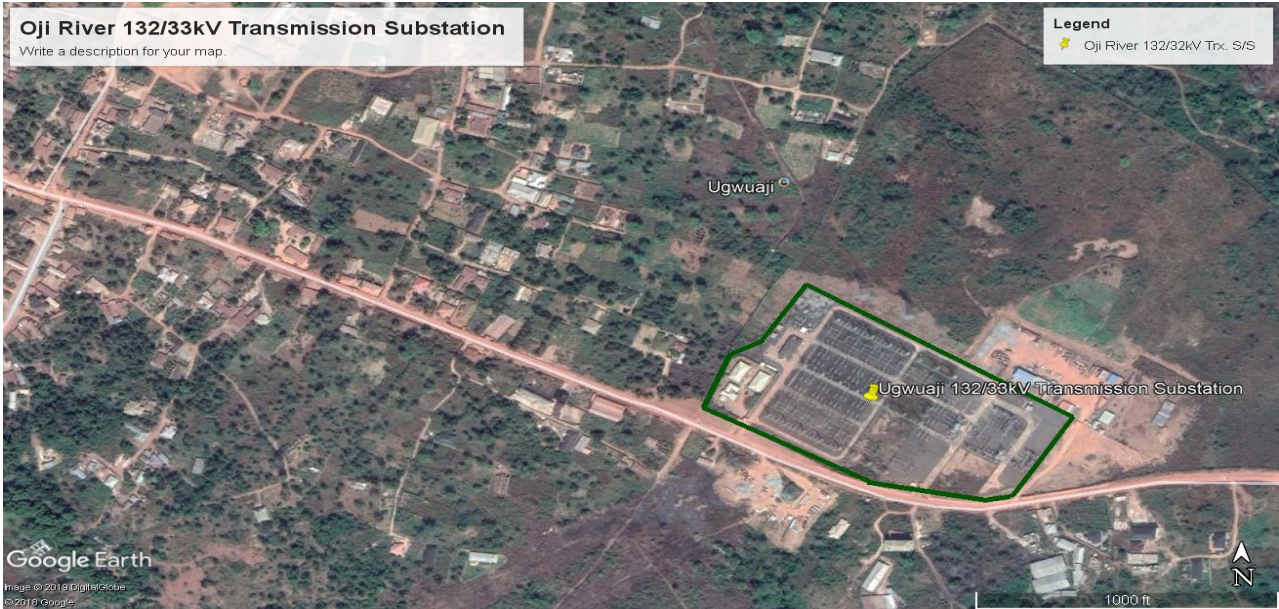
Figure 13: Satellite image showing Ugwuaji 132/33kV Transmission Substation.
