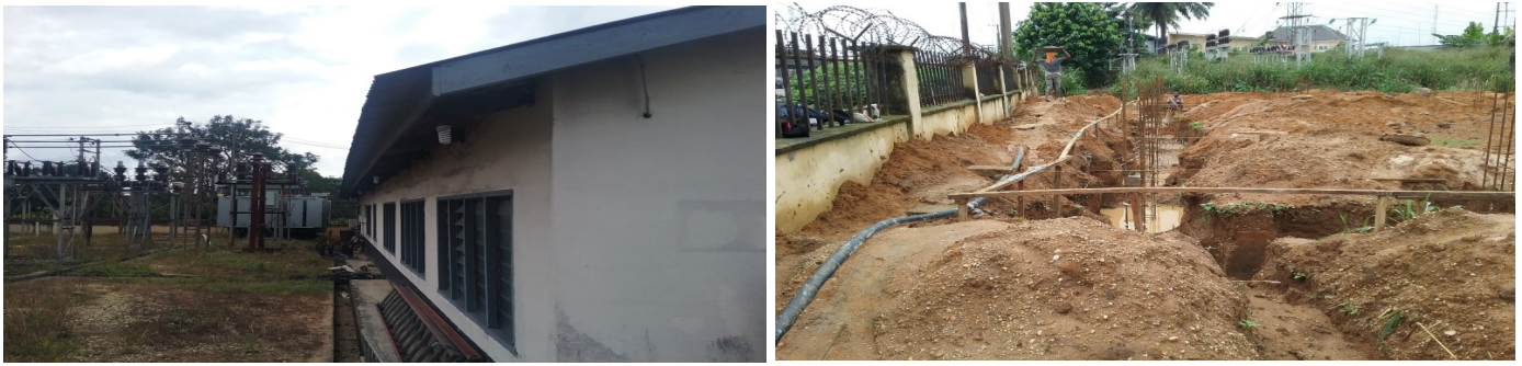
Figure 28: Existing Substation Control Room/ Foundation for new Control Room (under NEGIP).
