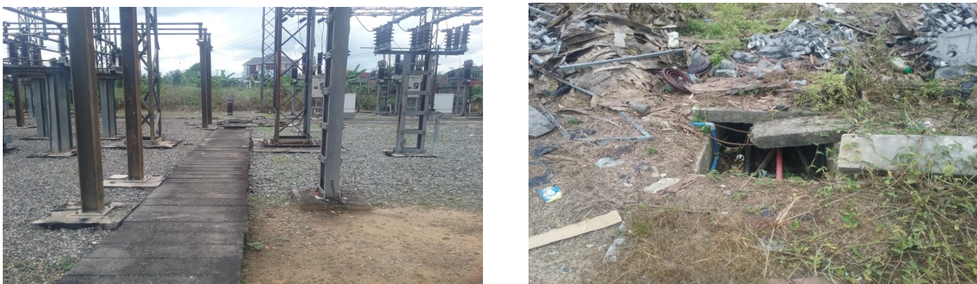
Figure 21: Sparsely graveled switchyard floor (with patches of light overgrowths)/ Exposed drainage cable trench.
