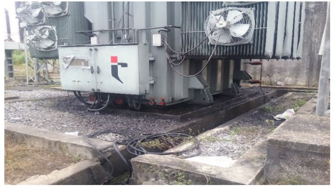
Figure 26: Blocked drainage channel resulting from sedimentation/Spilled oil at base of transformer.
