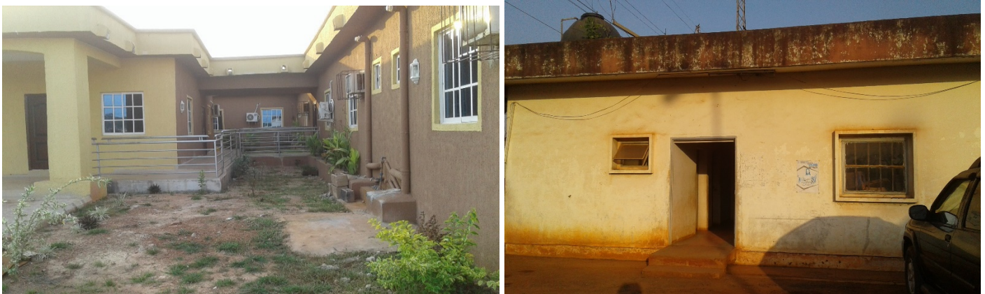
Figure 17: Substation Administrative building/Existing Control Room building.
