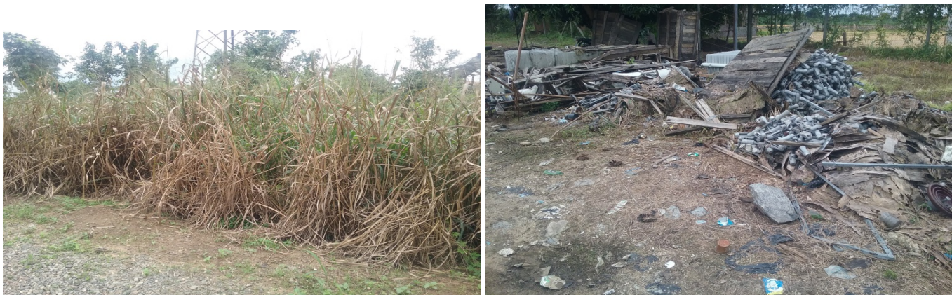
Figure 20: Dense Overgrowths within the Substation premise/Indiscriminate waste disposal within the substation.
