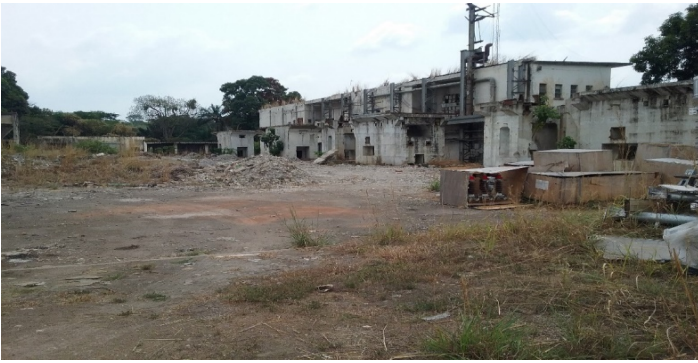
Figure 50: Very old and dilapidated building structure housing the Control Room for the Substation.
