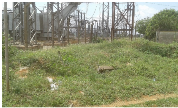
Figure 42: Poor storage of unused construction accessories/Dense Overgrowths within Substation premise.
