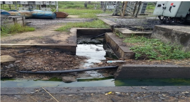
Figure 27: Spilled transformer oil trapped in stagnated water body (seepages have already affected the ground water supply).
