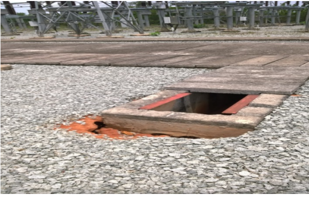
Figure 39: Erosion threat within the switchyard/Installation materials (from an on-going Project) in the switchyard (exposed to the vagaries of elements of weather and thefts).
