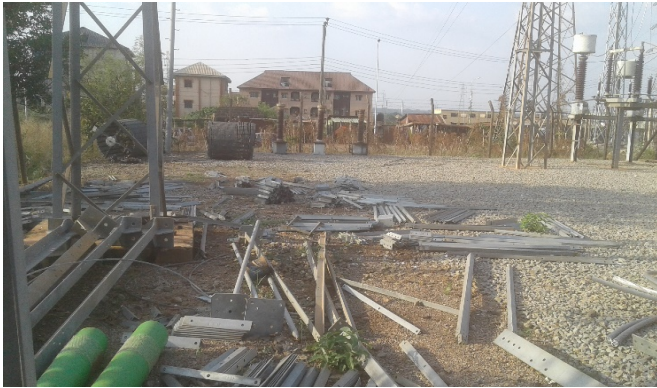
Figure 42: Poor storage of unused construction accessories/Dense Overgrowths within Substation premise.
