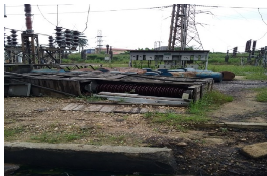
Figure 24: Decommissioned equipment littering the Substation premise/Poor storage of Construction Materials.
