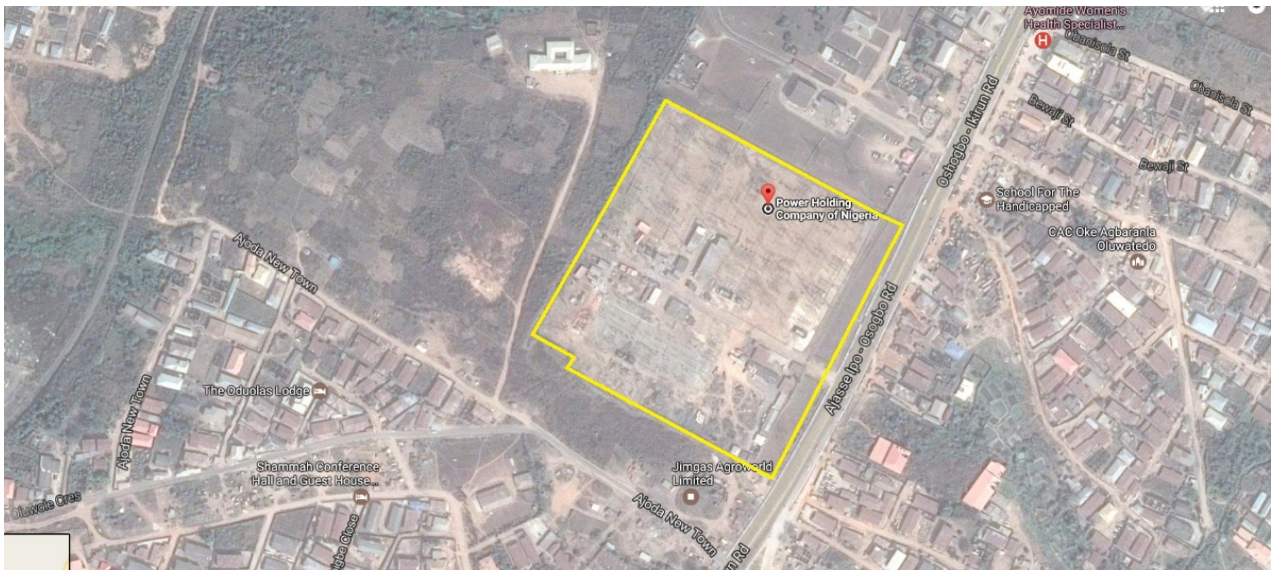
Figure 2: Satellite image showing Alaoji 330/132/33kV Transmission substation.
