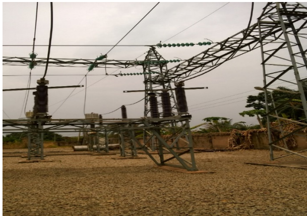
Figure 54: Properly maintained Switchyard floor
