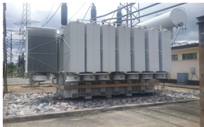
Figure 22: Weed growth in drainage channel/Oil Spill-free transformer base.
