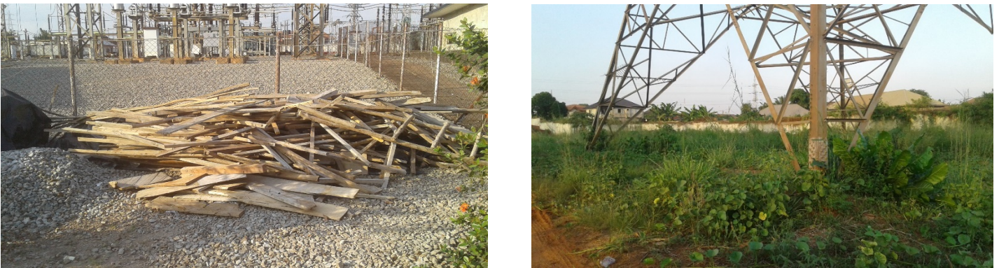
Figure 19: : Improperly disposed construction waste/Overgrowths within substation premise.
