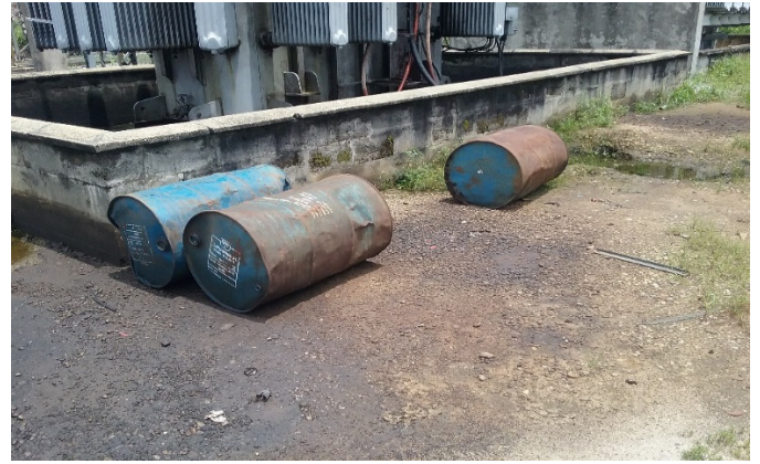
Figure 32: Overgrowths within the Substation premise/Improperly stored transformer oil drums.
