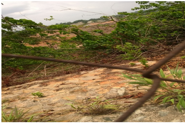
Figure 38: Excavation activities on-going Outside the substation.
