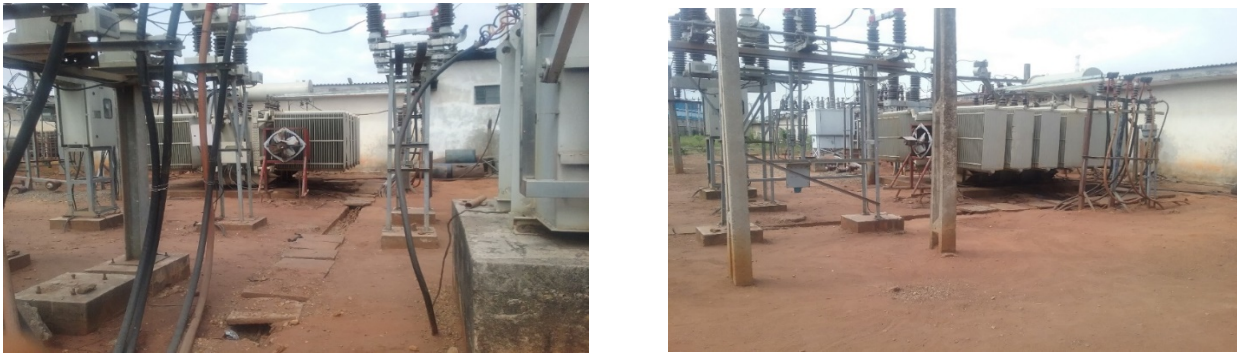
Figure 44: Blocked drainage channel resulting from sedimentation/ Switchyard properly maintained
