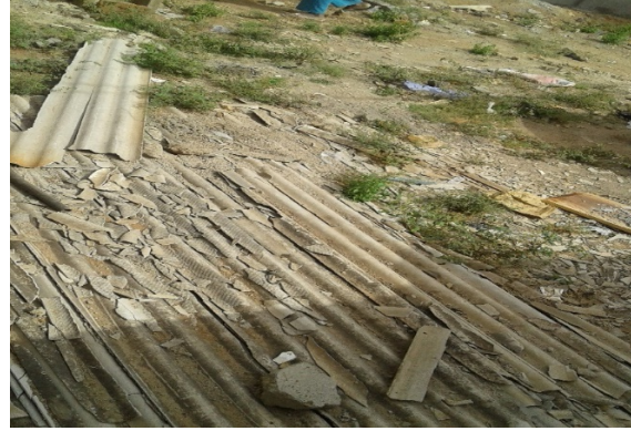
Figure 48: Scantly gravelled Switchyard floor/Scrap (asbestos) generated from on-going Rehab works at the Substation.
