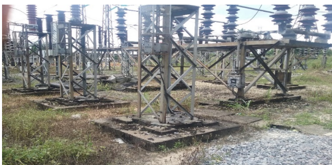
Figure 25: Overgrown weeds covering a significant part of the scantily graveled Switchyard floor/Overgrown weeds blocking drainage channels.
