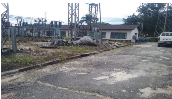
Figure 24: Decommissioned equipment littering the Substation premise/Poor storage of Construction Materials.
