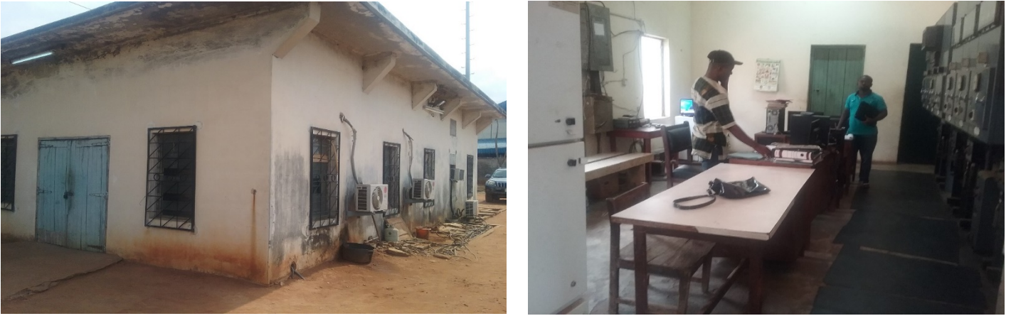
Figure 46: Very old and ill-maintained building structure housing the Substation Control Room/Decrepit furniture being use by operators.
