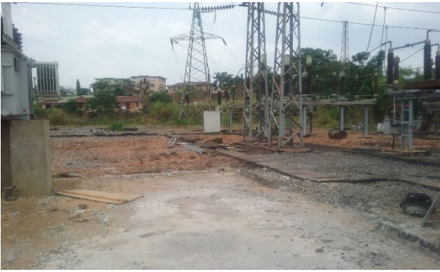
Figure 48: Scantly gravelled Switchyard floor/Scrap (asbestos) generated from on-going Rehab works at the Substation.
