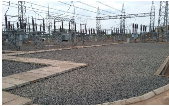
Figure 51: Properly maintained Switchyard floor/(well- gravelled and free of grasses or shrubs)/ Trench cover slabs intact, protecting power cables (eliminating the risks of accidental shock/electrocution).
