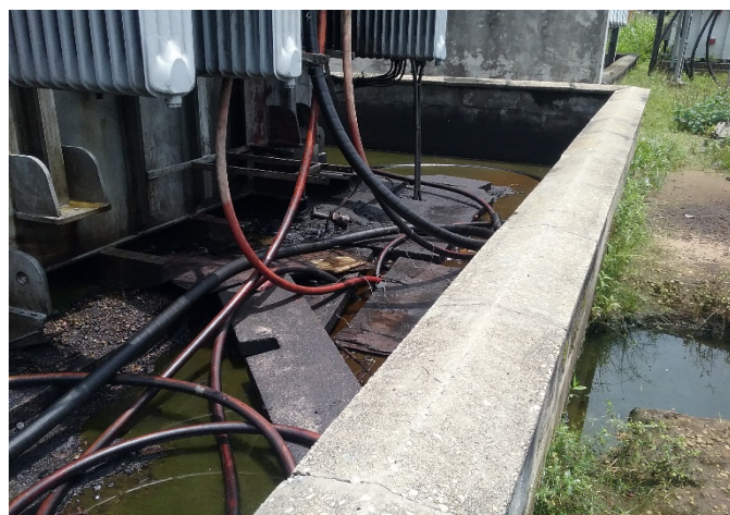
Figure 35: Transformer Plinth/Spilled oil from very old transformer(posing risks of ground-water pollution through seepage).
