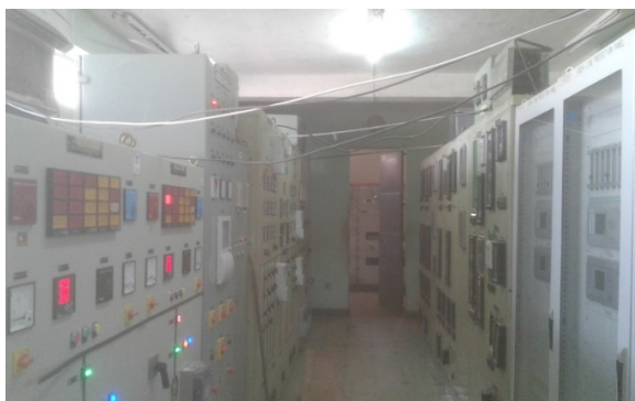
Figure 43: Control Panels in the Control Room/Working area within Substation Control Room.
