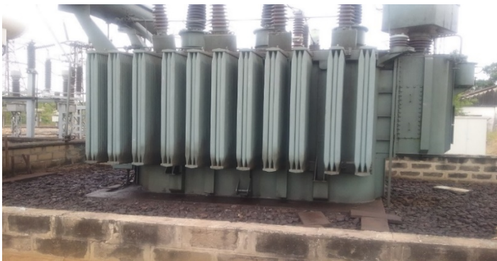
Figure 49: Oil leakage at transformer base.
