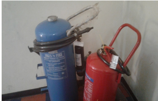
Figure 19: Fire Extinguishers at the Substation
