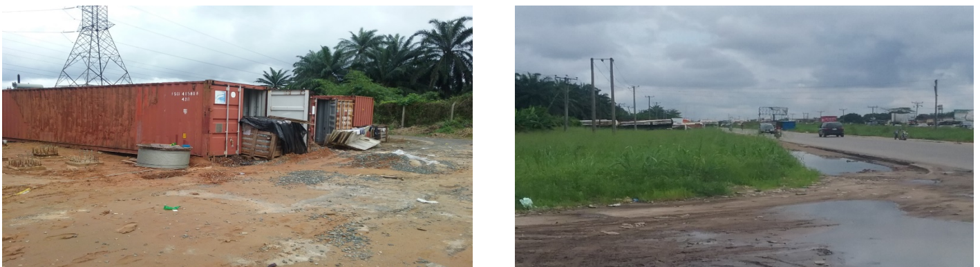
Figure 15: Containers used for storage of construction materials/Port Harcourt-Aba Road (leading to the Substation entrance).
