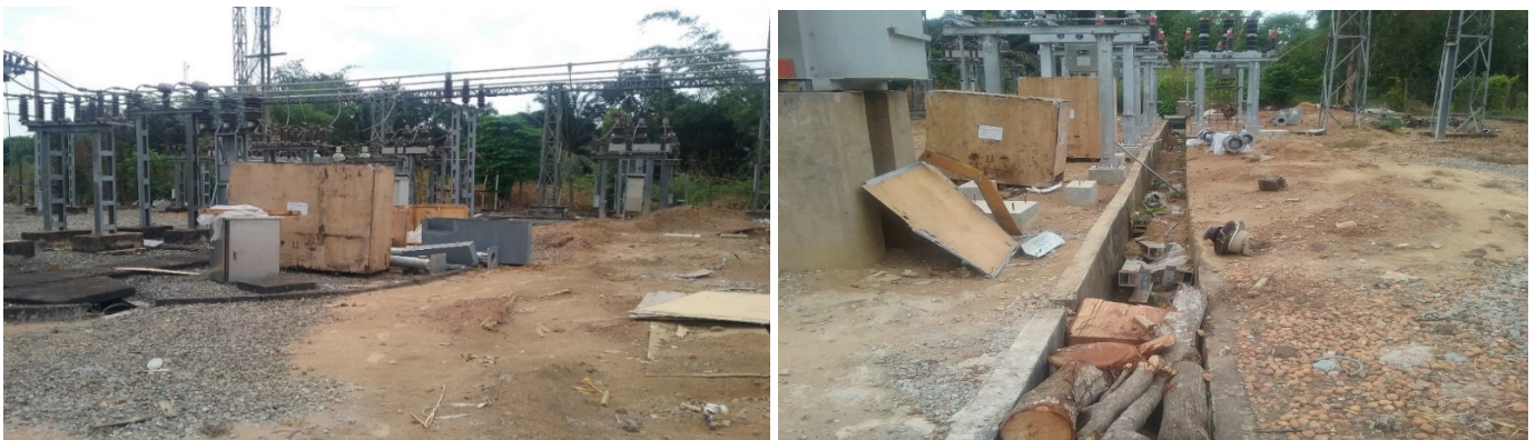
Figure 47: Equipment/materials and wastes littering the Substation premises/Blocked drainage channel resulting from sedimentation and dumping of waste.
