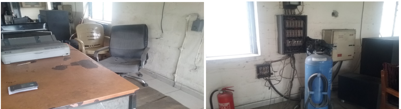
Figure 29: System Operators' Work area in the existing Substation Control Room/Fire extinguisher in Control room.
