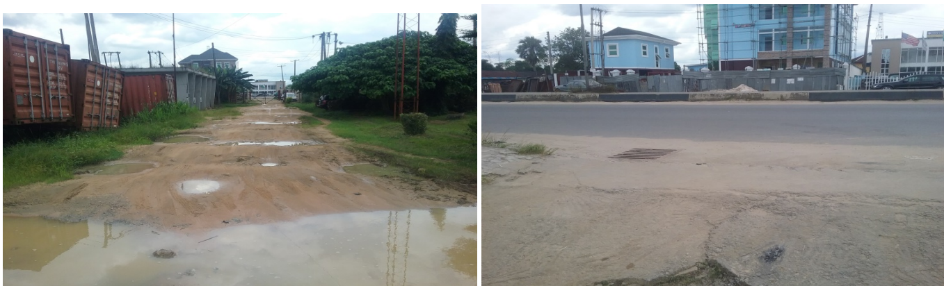
Figure 21: Drive path within Substation premise/Rumuobiokani Road (leading to the Substation entrance).
