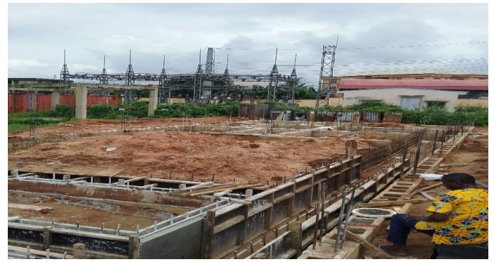
Figure 36: Exposed cables in the Control Room blocking run-off along the cable trench/Foundation for new Control Room Building being laid.
