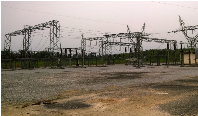
Figure 30: Itu 132/33kV Substation Switchyard/Existing 1x60MVA Transformer (No oil spillage noticeable)
