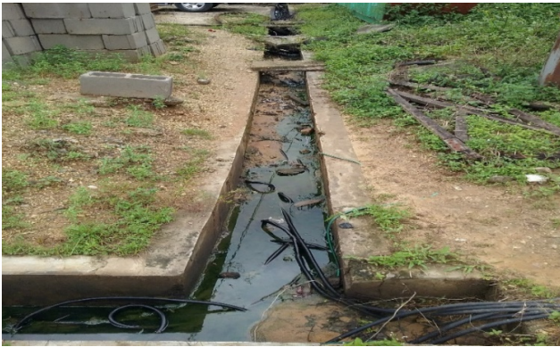
Figure 26: Blocked drainage channel resulting from sedimentation/Spilled oil at base of transformer.
