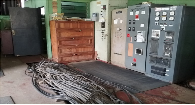
Figure 36: Exposed cables in the Control Room blocking run-off along the cable trench/Foundation for new Control Room Building being laid.
