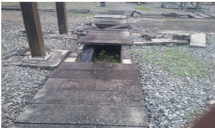
Figure 22: Weed growth in drainage channel/Oil Spill-free transformer base.
