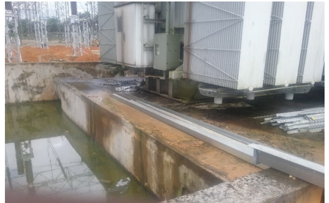
Figure 16: Properly maintained switchyard floor/Stagnated water body at base of transformer.
