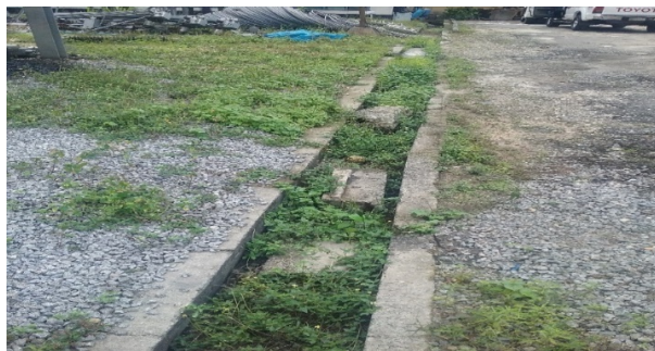
Figure 25: Overgrown weeds covering a significant part of the scantily graveled Switchyard floor/Overgrown weeds blocking drainage channels.
