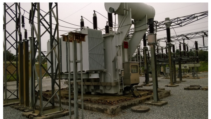
Figure 30: Itu 132/33kV Substation Switchyard/Existing 1x60MVA Transformer (No oil spillage noticeable)
