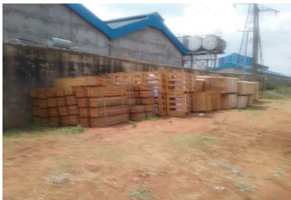
Figure 45: Construction materials neatly stacked but unprotected (leaving them susceptible to degradation, defectiveness or theft).
