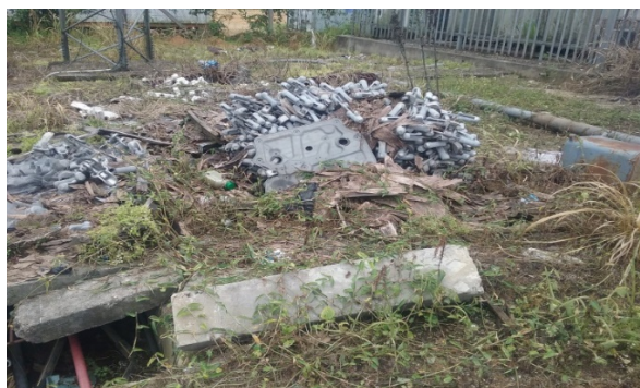
Figure 23: Improperly stored accessories strewn on the Substation premise/Indiscriminate waste disposal within the Substation premise.
